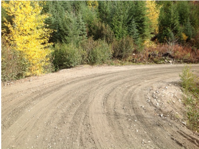
Approach from Right Bank when facing downstream
